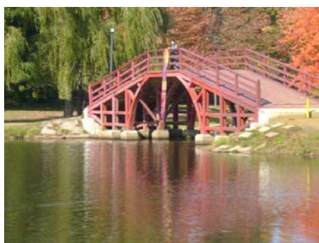
Red Wooden Bridge
